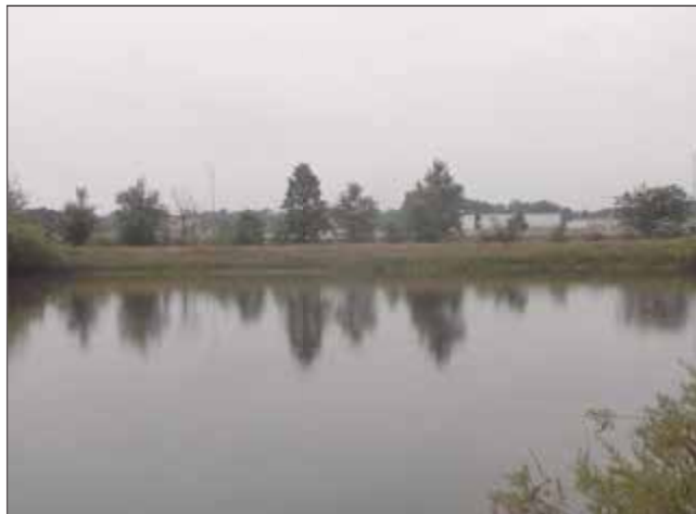
PHOTO 5: View of Detention Basin 1 facing northeast. Photo date: 8/18/2015
