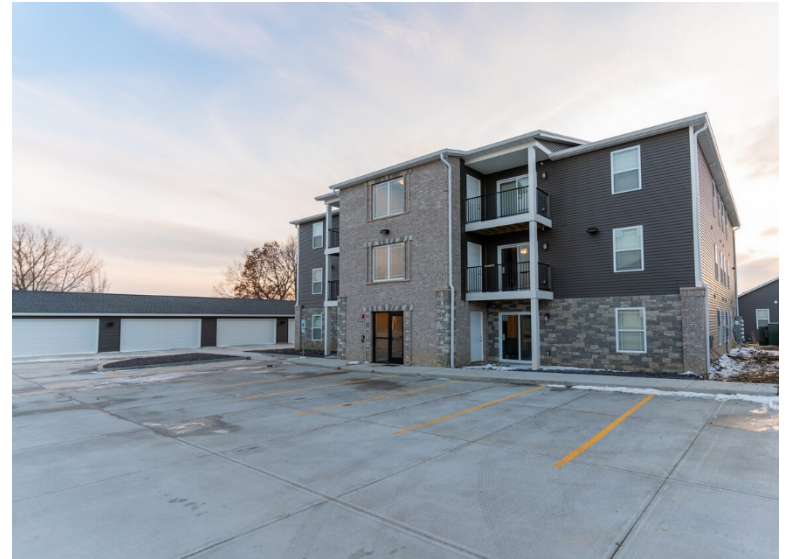
The Crossing Apartments
