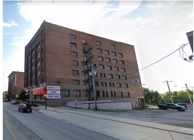
812 Lofts (Under Construction)
