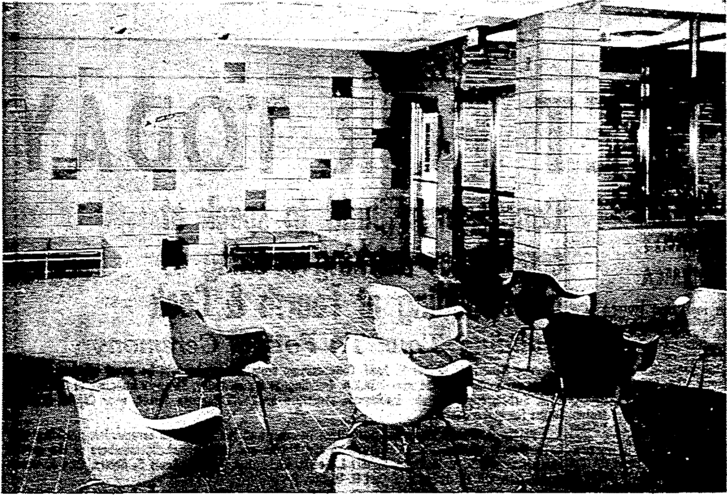
Boys will be boys, but in spite of heavy traffic, this wall, being scuff resistant and virtually dust free, will require only infrequent cleaning. Arketex ceramic glazed structural facing tile is shown above in the main lobby youth entrance.
