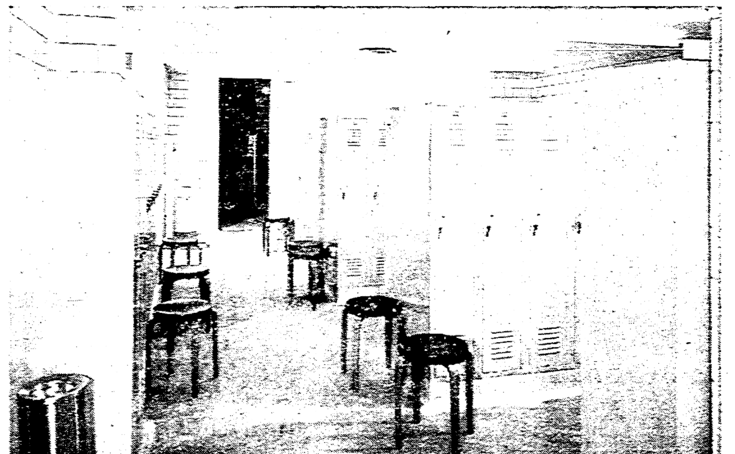
Many of the visitors to the dedication and open house will see and admire the expanded locker room facilities. The work of one contractor will not be shown, although it is vital to the building and contents . . . the roof. The roof was installed by Schmidt Bros., Inc. Electric circuits and lighting were installed by Volie Electric Service.
