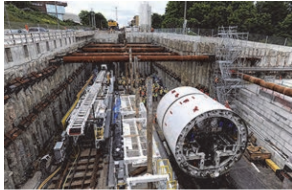
The tunnel-boring machine at the Eglinton Crosstown LRT construction site.
