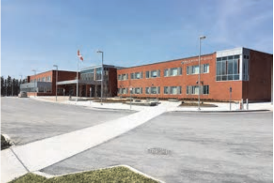
Orillia Secondary School opened in March 2016.
