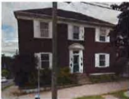
Simplified Cornice (no dentils or corbels)
