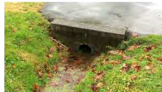
Storm Sewer - $165,000 Loc Improvement, Misc
